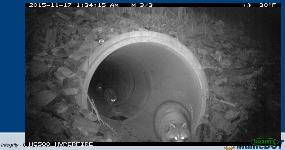
1.4 (54 inch) high culvert with concrete pad as shelf winter use (Cameras at each end have shown through passage)
